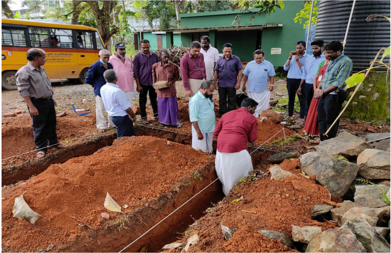
Photo.2 Sri.D.Rameshan (Kattaikaonam,Councilor) laying foundation stone
