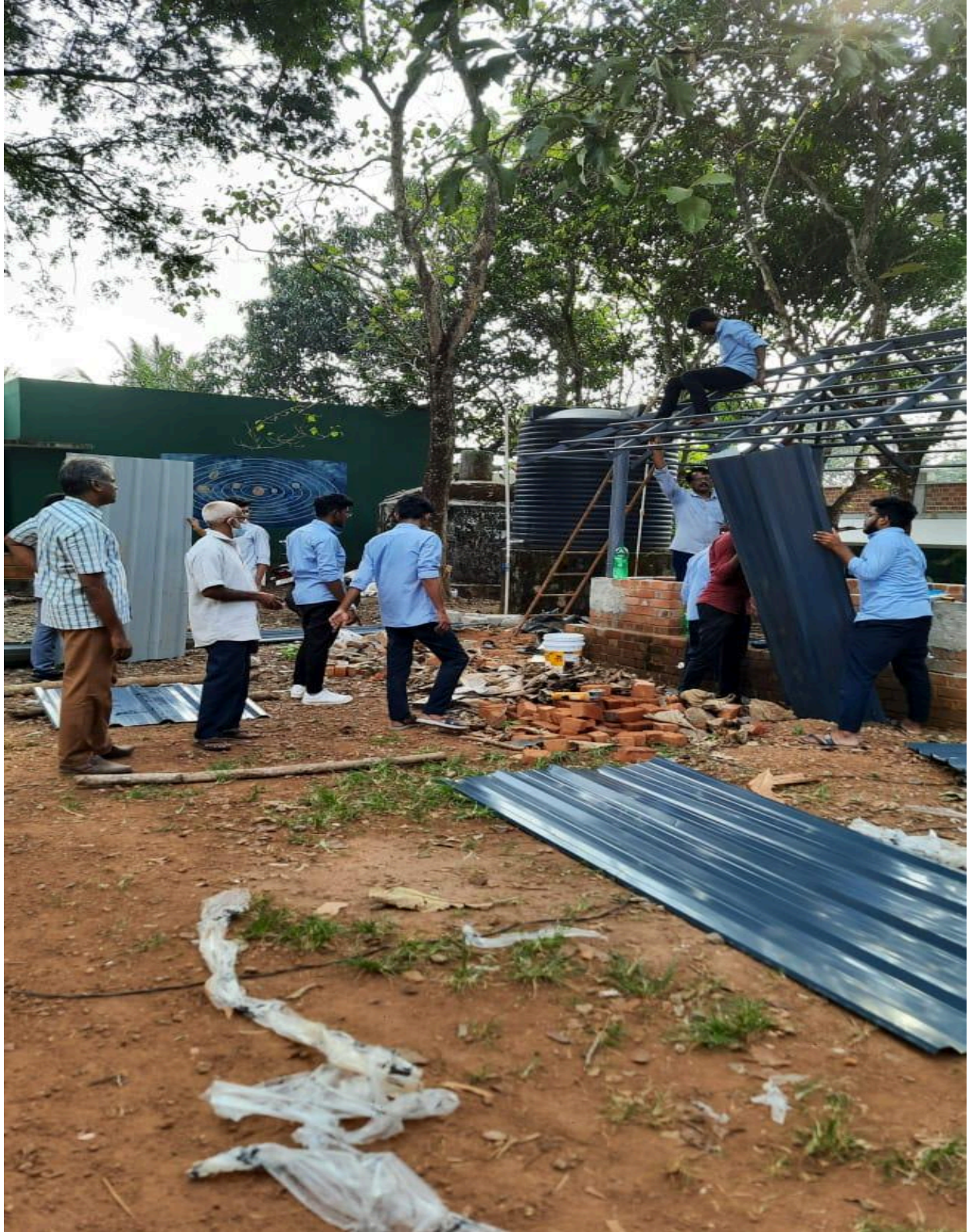
Photo.6.Roof GI sheet (JSW COLOURON)laying in progress
