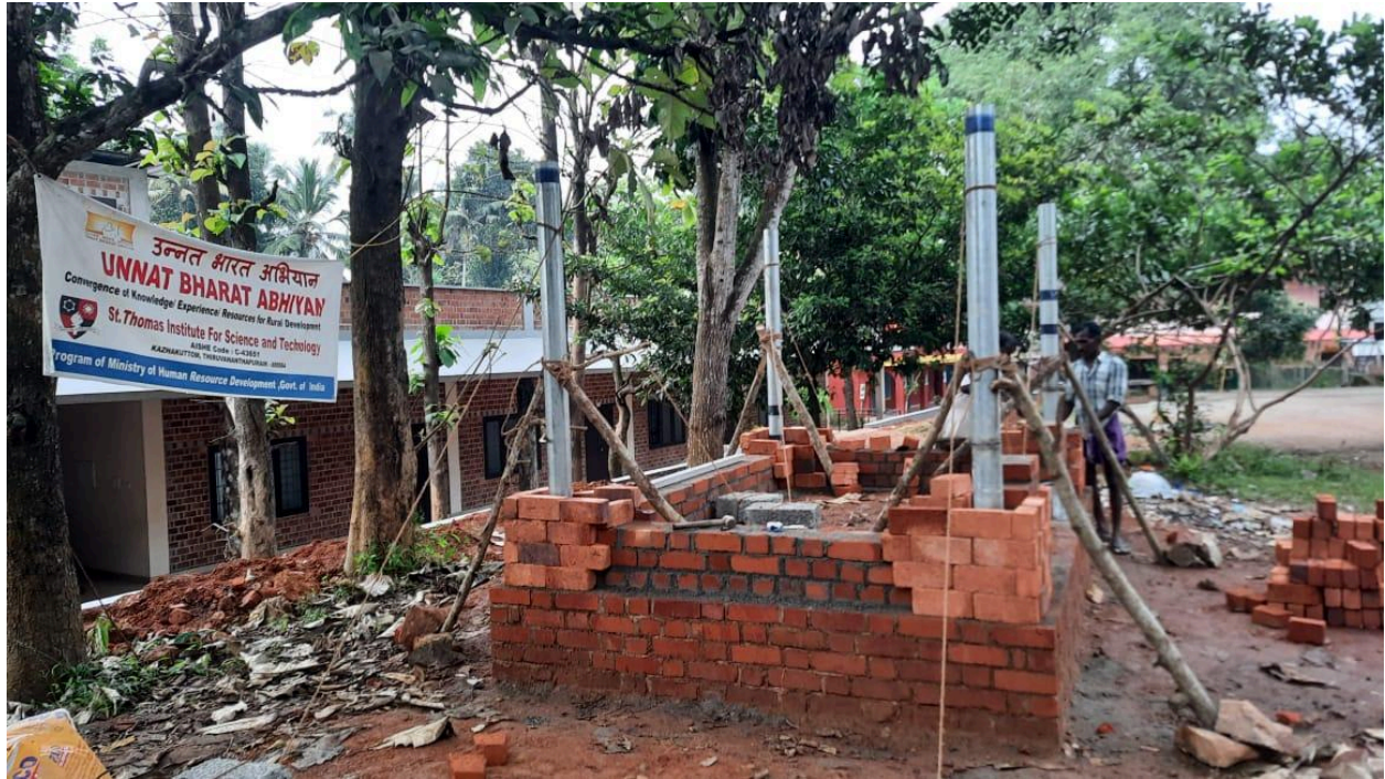
Photo.4 Four G.I circular pipes installed for roof support
