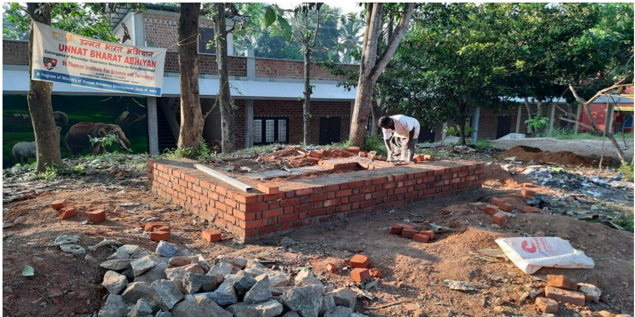
Photo.3 Bricklaying in Progress
