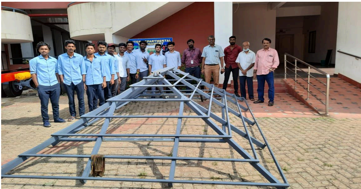
Photo.5 .Roof frame welding completed with GI circular & rectangular pipes in STIST workshop
